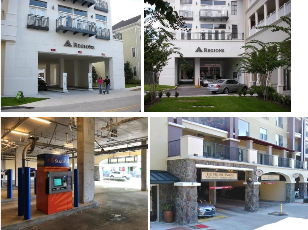
Figure VIII - 44. Interior Drive-Through Facilities
