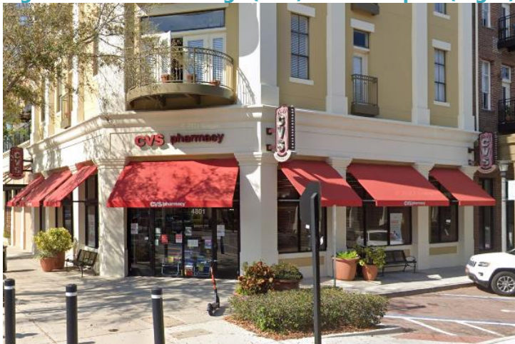
Figure VIII - 23. Awnings (Left) and Canopies (Right)
